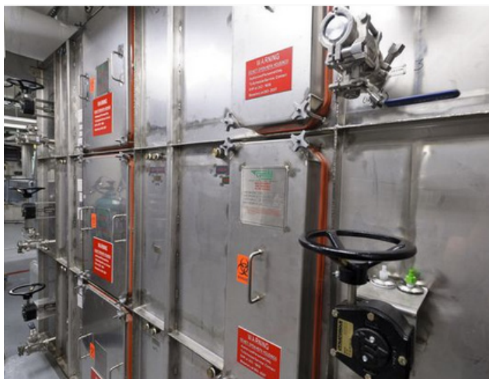
A ventilation system designed to filter the building's air supply through a series of HEPA filters is seen during a tour of the Influenza Research Institute at the University of Wisconsin-Madison on Feb. 13, 2013.
